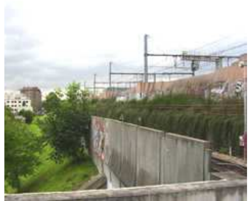
Talus SNCF RATP
